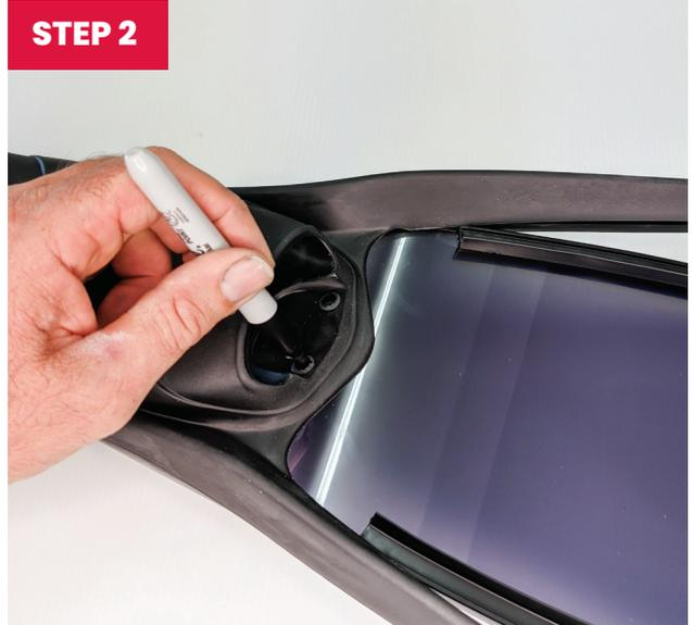
Mark position of the fixing kit holes with a permanent marker. These will be a guide for drilling the holes.
