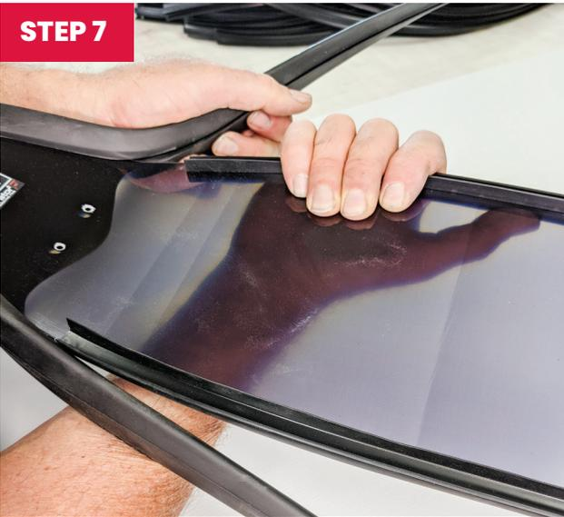
Push the blade all the way into the pocket until screw holes align with the holes in the pocket.
